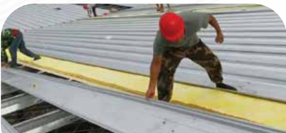
CLASS WOOL SHEET LAYING
