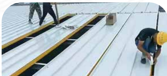
PUF PANEL FIXING
