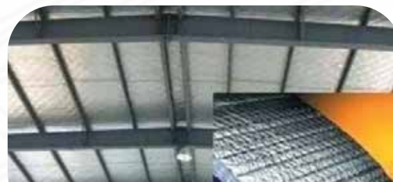
XLPE INSULATION SHEET FIXING
