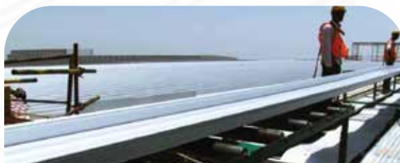
PRODUCTION OF STANDING SEAM SHEETS
