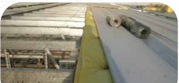
ROCKWOOL SHEET LAYING
